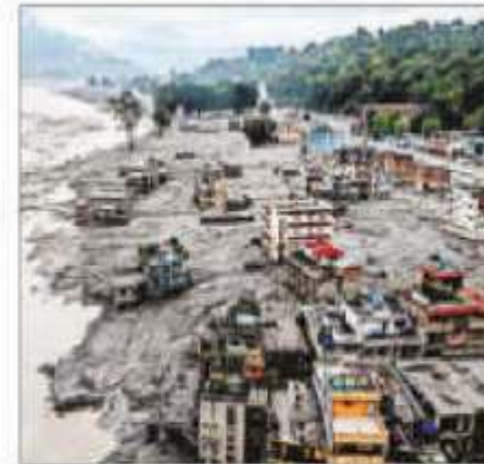
Drone view shows mud-covered buildings after flash floods in Devighat, Nepal. FILE
