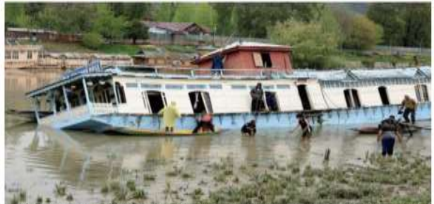
Rain impacts: People attempt to salvage a damaged, partially repaired boat along the banks of the Jhelum River in Srinagar, Jammu and Kashmir, following rain on Wednesday. istat news
