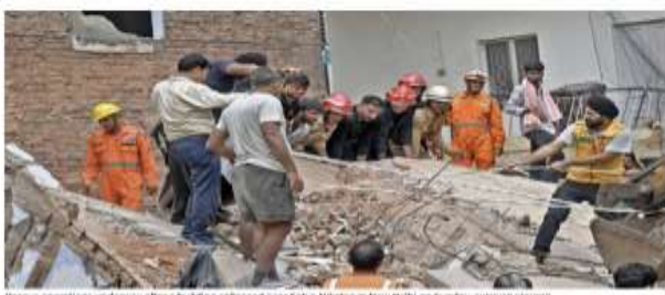
Rescue operations underway after a building collapsed near Safa Nigrah in New Delhi on Sunday. • ANI/PTI
