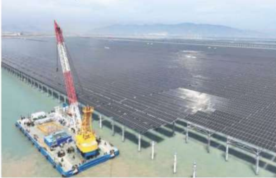
Towards sustainability: Solar panels being placed at the CNNC Tianwan tidal flat photovoltaic power plant in Lianyungang, in China's eastern Jiangsu province, on April 19.
