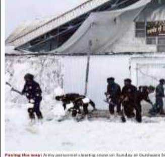
Paving the way: Army personnel clearing snow on Sunday at Gurubandh Sri Hanuman Sahib in Chameli district of Uttarakhand, ahead of its opening. The Hanuman Sahib yatra begins on May 21. PPT
