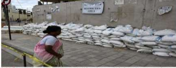
Beated off: A notice has been placed declaring the area restricted following the compound wall collapse at the government-run Borewing and Lady Caxson Hospital in Shivajinagar, Bengaluru, on April 29, 2020. L.A.S.R. SIDDHANTH
