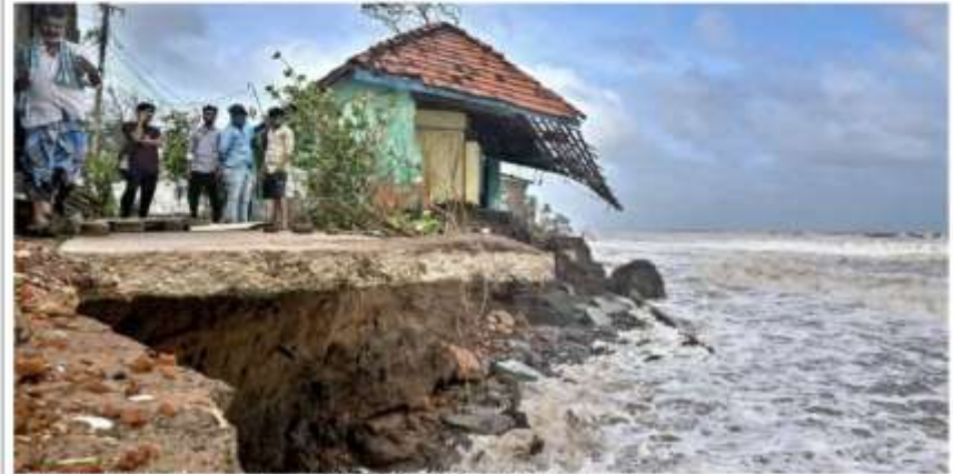
Swept away: A home destroyed by the cyclonic swell in Kakina district of Andhra Pradesh on Tuesday. K.A. DEENA
