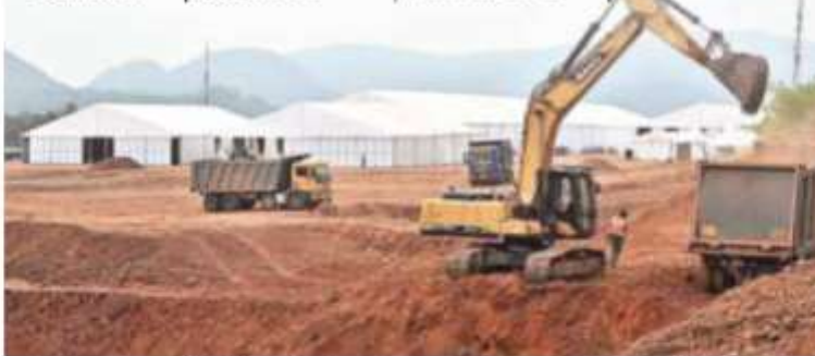
Arrangements in full swing for the stone-laying ceremony of Google Data Centre at Tarluvada, a suburban area of Visakhapatnam. V. RAJU
