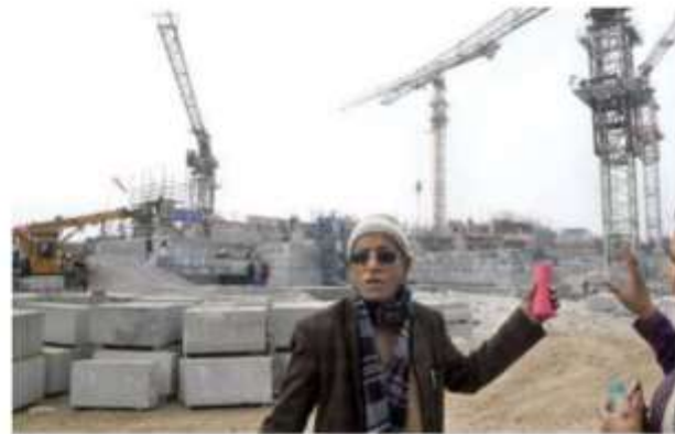
Champat Rai, chief of the temple trust, during the construction of the Ram Temple in Ayodhya in January 2023. SANDEEP SAXENA
