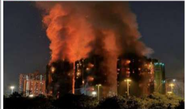
A fire engulfed several apartment blocks at the Wang Fui Court residential estate in Hong Kong's Tai Po district on Wednesday, killing at least 30 people and leaving more than 200 unaccounted for in the city's worst blaze in decades, air police say.
