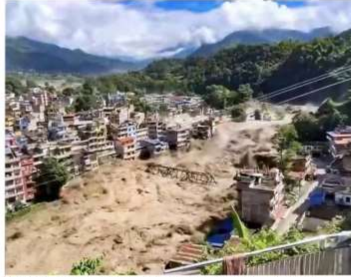
Flood fury: A screenshot shows water flowing across a residential area and damaging a bridge near the Nepal-Tibet border. (1)
