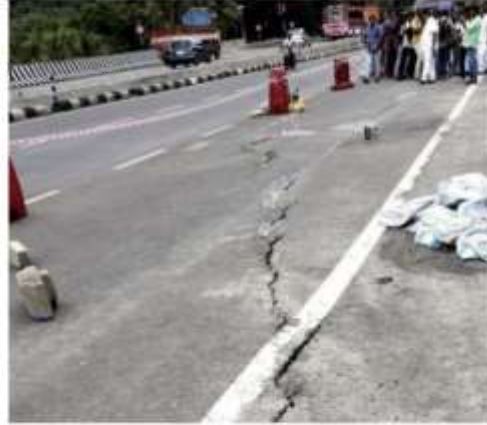
Data on the status of roads shall be collected for all projects involving two- to eight-lane highways. FILE PHOTO
