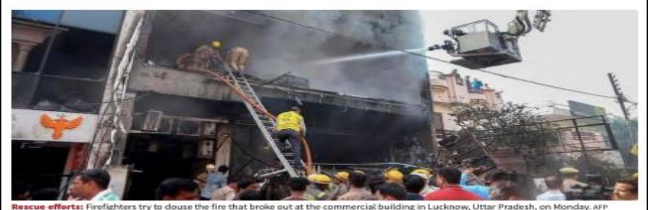
Rescue efforts: Firefighters try to douse the fire that broke out at the commercial building in Lucknow, Uttar Pradesh, on Monday. AFP
