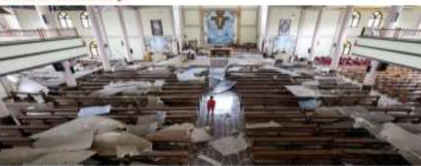
A child stands inside the damaged St. Francis Xavier Church, in the aftermath of an earthquake, in Buring, Mangrove region, Indonesia, on Monday. The 7.7 magnitude quake on Saturday has left at least 64 people and 1,300 displaced. AP
