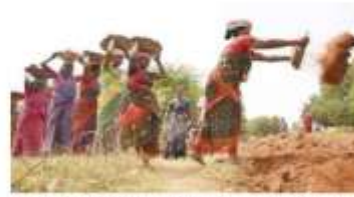
Hard labour: MGNREGS beneficiaries widen a supply channel at a work site in Sivaganga district of Tamil Nadu. MOONRI G.
