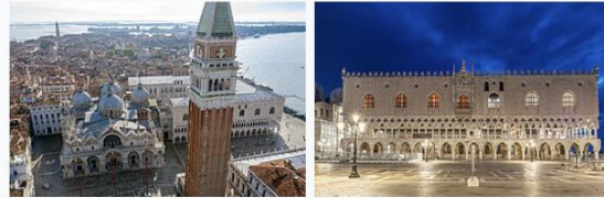
St Mark's Campanile
