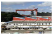
CSL became the third shipyard to enter into a pact with the U.S. Navy, which will enable to repair U.S. Navy ships. The State-run shipbuilding facility in Kochi is the latest in the line after Larssen Offshore (L&T) and Mazagon Dock Shipbuilders Ltd. (MDL).
