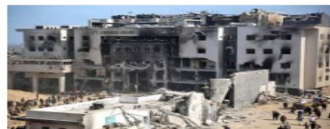
Dilapidated state: Palestinians inspect the damage at Gaza's al-Shifa hospital after the Israeli military withdrew on Monday. AFP
