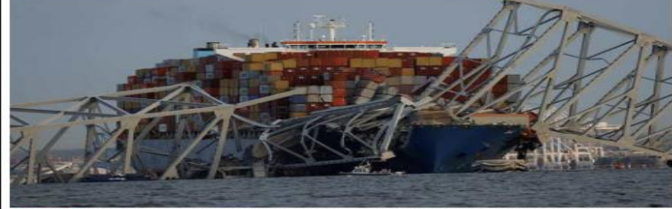
Brought down! The Francis Scott Key Bridge over the Patuxent River at Baltimore, U.S., which caved in after a cargo vessel with an all-Indian crew crashed into it on Tuesday. At least 7 people have gone missing in the incident. REUTERS (REPORT ON PAGE 14)
