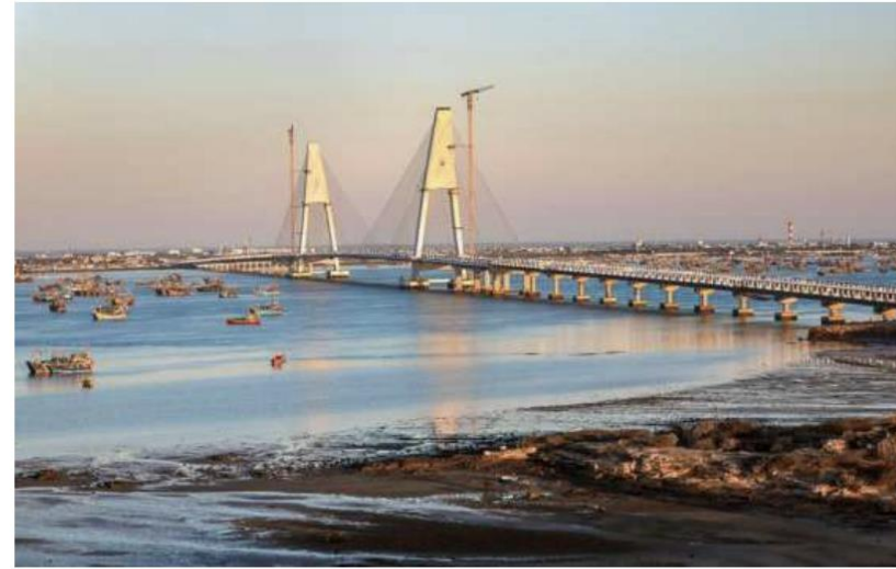
Grand launch: Sudarshan Setu, India's longest cable-stayed bridge that will connect Okha mainland and Beyt Dwarka island in Gujarat. Prime Minister Narendra Modi inaugurated the bridge on Sunday. PTI
