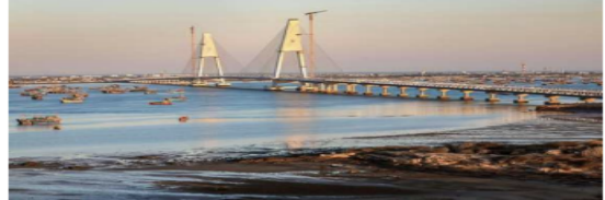
Grand launch! Sudarshan Setu, India's longest cable-stayed bridge that will connect Okha mainland and Bekt Dwaraka island in Gujarat. Prime Minister Narendra Modi inaugurated the bridge on Sunday. PPT
