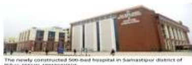
The newly constructed 500-bed hospital in Samastipur district of Bihar.
