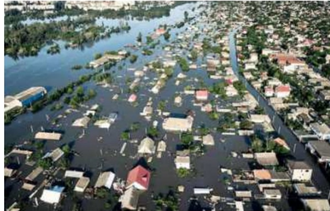
Brink of disaster: Flooded streets in Kherson on Wednesday after the walls of the Kakhovka dam collapsed. AP
