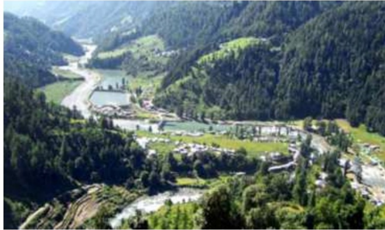
A view of the Shanan hydroelectric power project in Himachal Pradesh's Mandi. SPECIAL ARRANGEMENT
